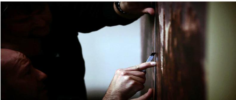
9) Using a sharp knife, cut through the middle of the overlapped layers (both layers) from top to bottom right through and then remove both of the small off cuts. The seams should now be perfectly clean.
